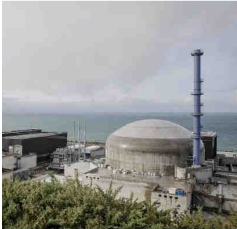
Figure 2: EPR dome at Flamanville, showing concrete patina. Photo copyright: Bloomberg
